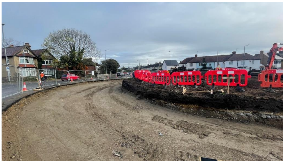
Work to remodel the roundabout is now underway
