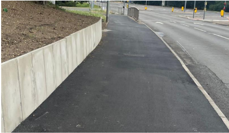
Pictures showing completed works at the Science Park
