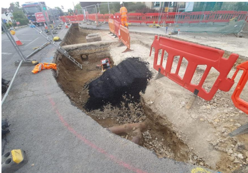
Excavation of works at Woodhead Drive.
