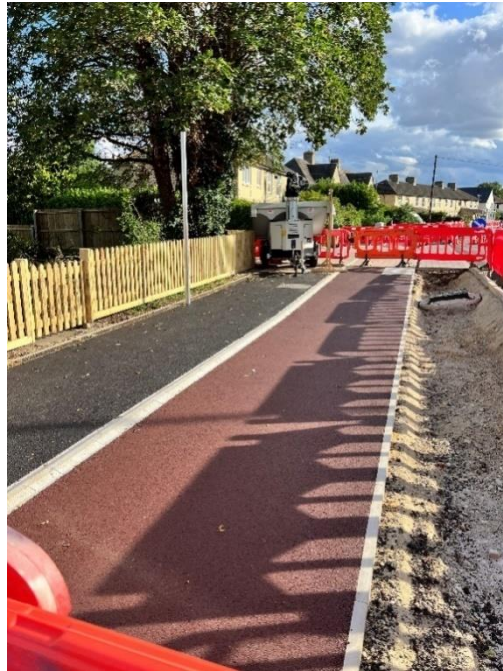
New cycleway and footway opposite Arbury Road shops.
