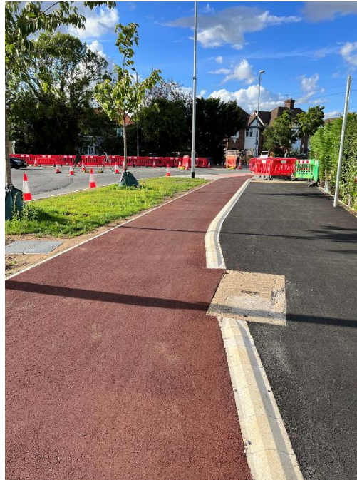
Completed northeast quadrant of Elizabeth Way roundabout.
