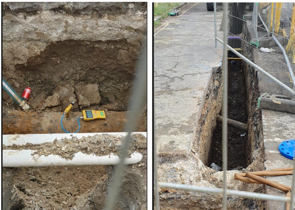
Pressure testing being carried out by Cadent Gas.
