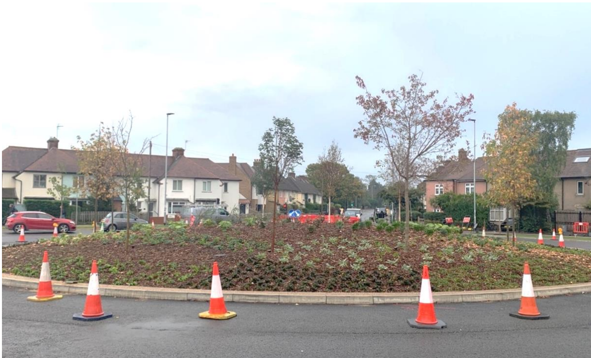
Completed landscaping at Highworth Avenue / Elizabeth Way roundabout
