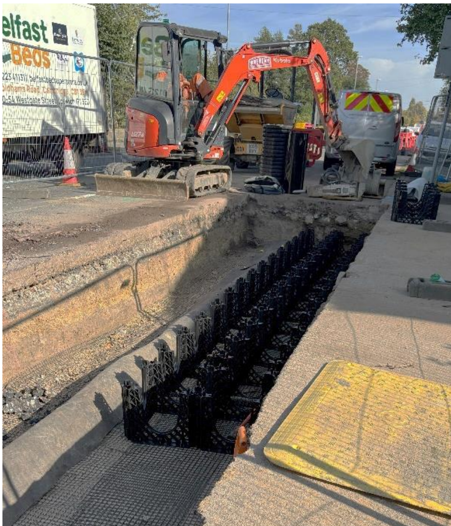
Tree pit and soil cell installation
